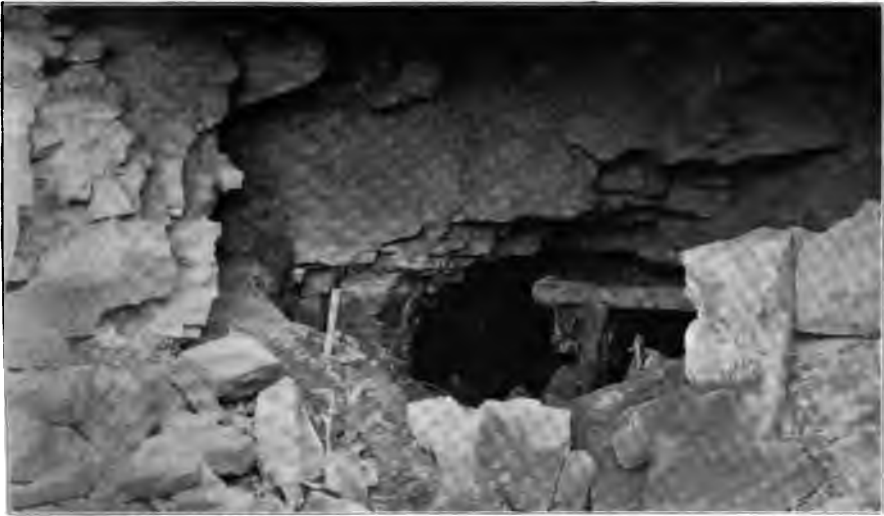
A.—A small drift mine in the Sharon or No. 1 coal on the north side of Chip-pewa Valley. Note the sandstone roof.
